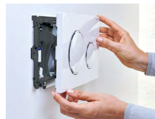
← It doesn't get any simpler than this: pull the actuator plate aside.
